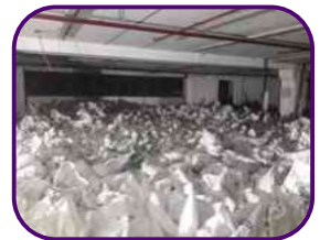
Slab Load Test
